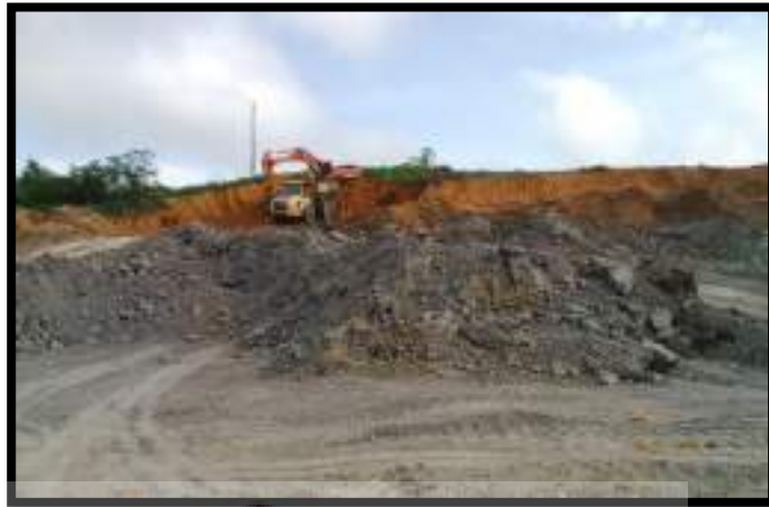
Gambar 4.3. Removal Top Soil
