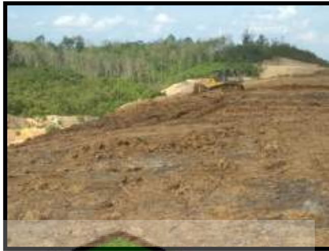
Gambar 4.5. Penebaran Topsoil
